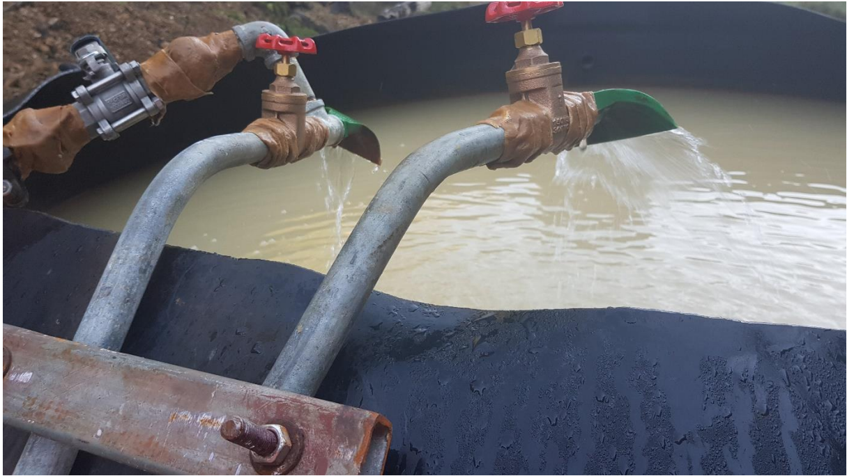
Figure 4.4-2: Photograph of the TSF water (right) and the RDRN influent water (left) entering the VFR through the spray nozzles.
