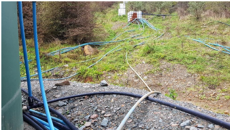
Figure 7: Photographs of samples and the operational bioreactors. A: Samples from the bioreactors; B: Effluent pipes from the bioreactors discharging into sump; and C: IBC feed tank with the inlet lines to the bioreactors.
