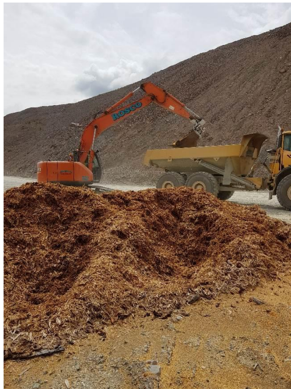
Figure 1. Photographs of the set up of the bioreactors. A: Underdrain pipes being covered with drainage gravel; B: Underdrain pipes being installed; C: Biosolids being delivered to load up area; and D: Truck being loaded with substrates.
