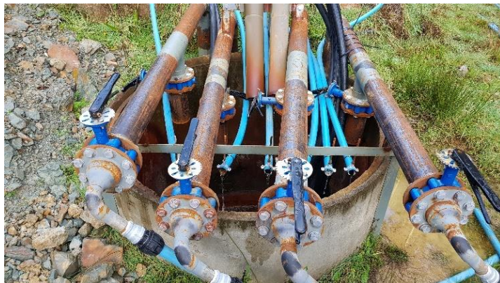
Figure 4.3-7: Photo of the seepage collection sump showing underdrain pipes (large metal pipes) transitioning into 40mm alkathene pipe being fed back up to the WRS to the feed IBC. Also, 40mm bioreactor outlets discharging into the collection sump.
