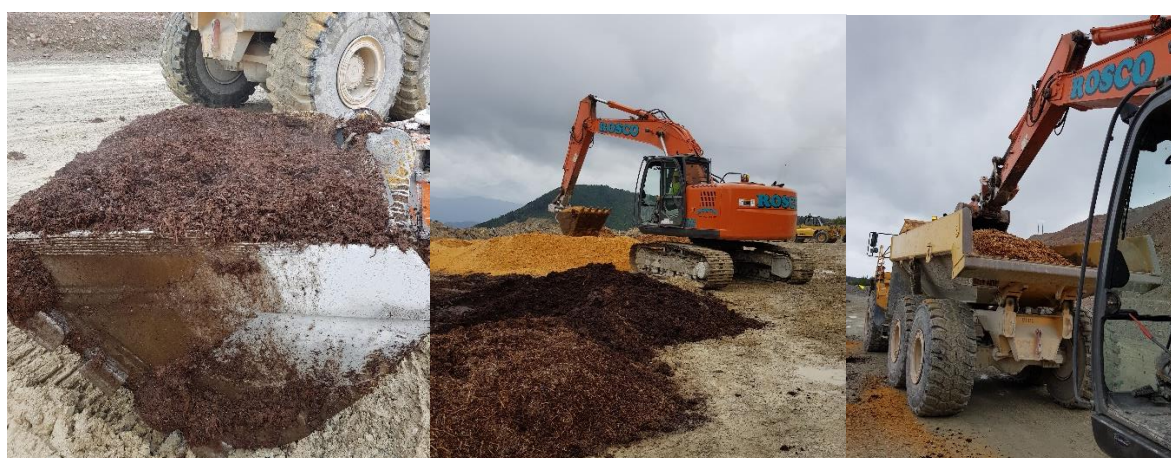
Figure 4.3-2: Photos of media being loaded and mixed. From left: 1) Bucket with SMC 2) Digger with bucket of sawdust 3) Digger mixing media in back of dump truck.
